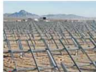
3 - Pose des structures de support.
